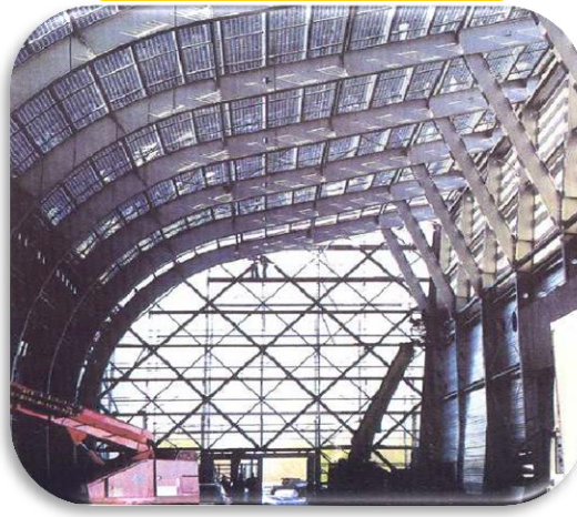
Special projects BIPV 100 kW
