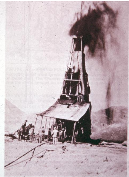
PLATE 3.1 A CABLE-TOOL GUSHER This photograph, taken in 1911, shows one of the very early company wells drilled on the "maidan" at Masjid-i-Sulaiman after penetrating the reservoir.
