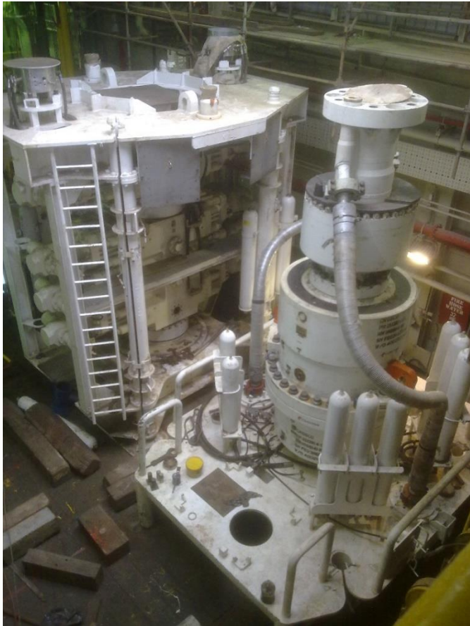
Source: INAgip, Plc photodocumentation;
