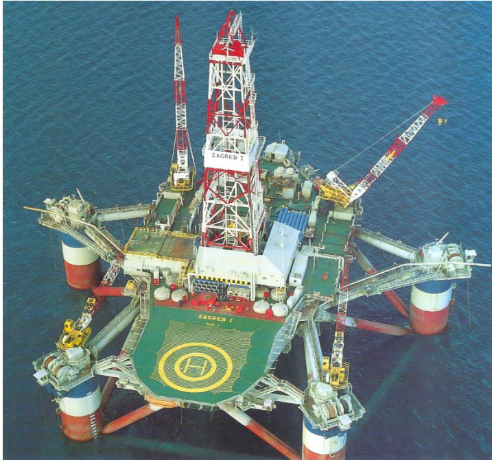
Semisubmersible drilling platform Zagreb - 1
