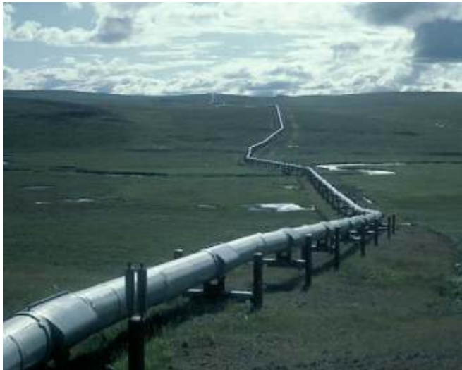
Natural gas pipeline
